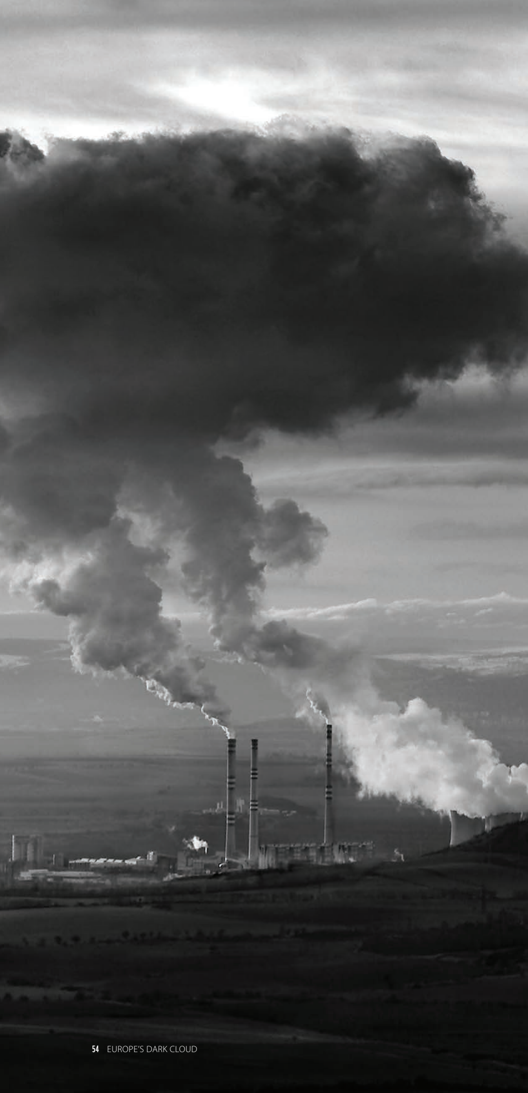
POČERADY POWER PLANT, CZECH REPUBLIC. © zahorec
