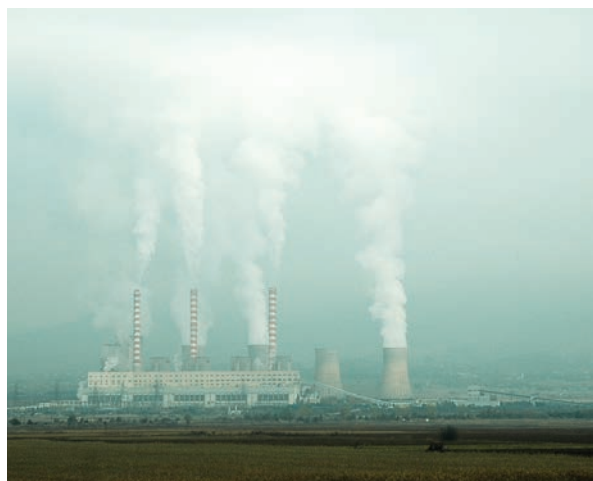
AGRIOS DIMITRIOS POWER PLANT. © Ioannis Tokaris
